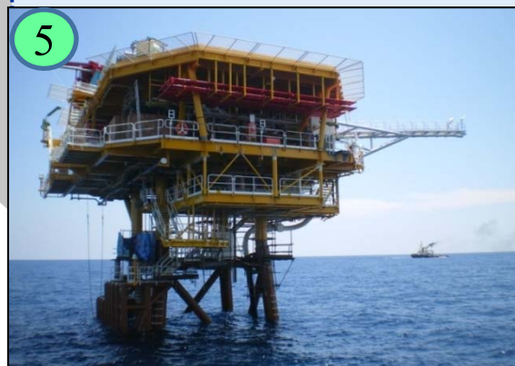
Example of installed platform
