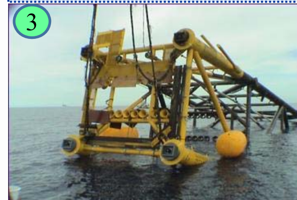
Installation of platform jacket
