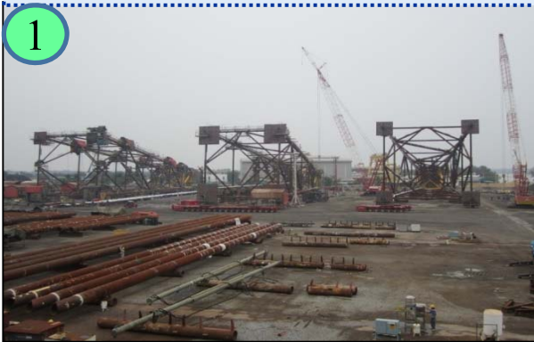
Platform structure assembled at onshore
