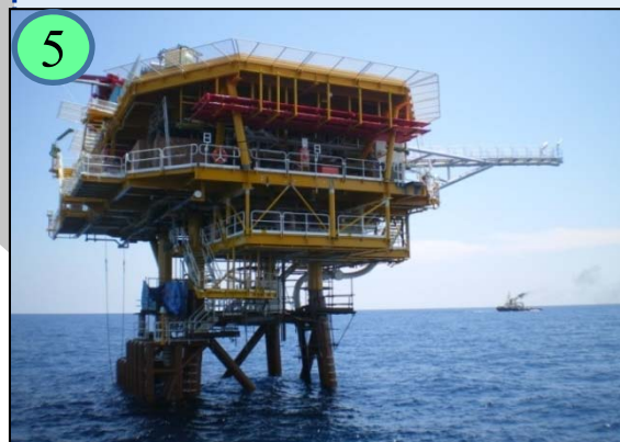
Example of installed platform
