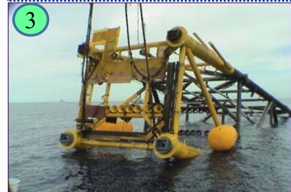
Installation of platform jacket
